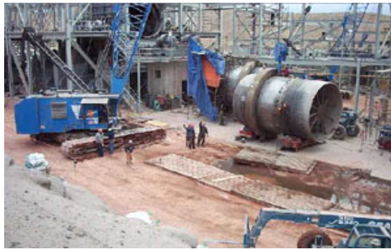
Additional installation time, maintenance, plant unavailability lead to a cost increase
