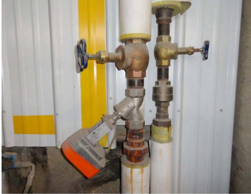
Figure 6. Wireless 4-20 mA control signal sent to steam valve.
