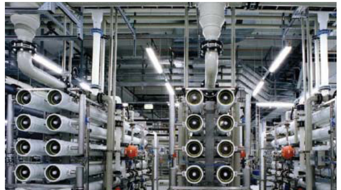
Reverse Osmosis Membrane Stack in Power Utility
